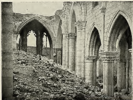
Cerny-les-Reims. Interior of the church, destroyed by the French artillery
